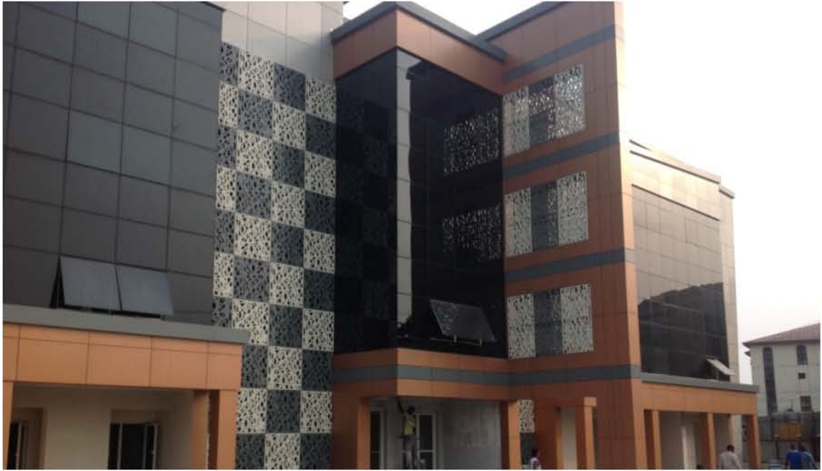
Port Harcourt, Rivers State Remodeling, Construction and Landscaping of Produce House
